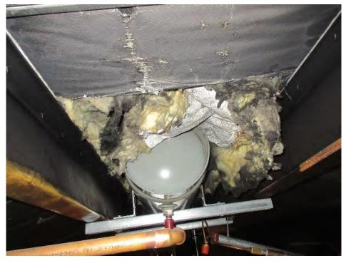
Figure 4: Damage to Interior Insulation of the Building due to Roof Leaks
