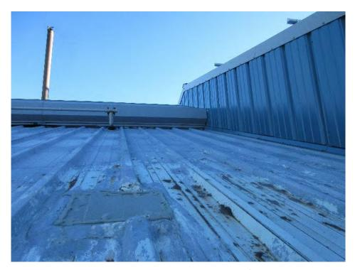
Figure 3: Large Section of Roof with Rusted Panels - Patching/Sealing has been Attempted
