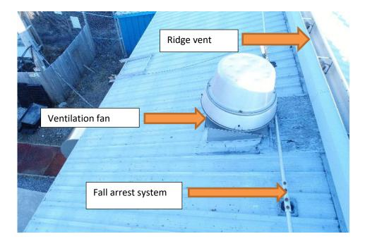
Figure 6: Exhaust Fan Hood (which has been patched around), Fall Arrest System, and Ridge Vent.
